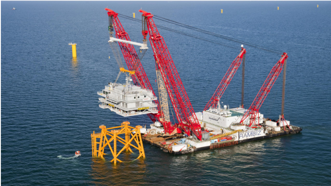
Figur 6. Heavy Lift Crane.
